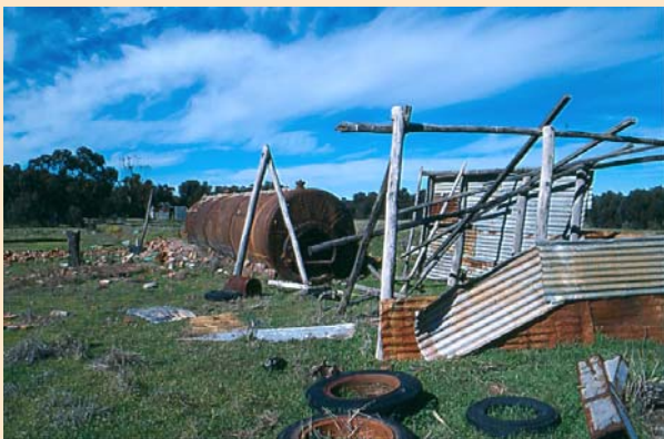
Campbell's eucy distillery boiler. Courtesy of DSE.
